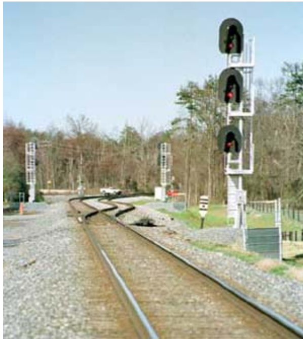
Figure 11: Control Point with Three Signal Heads
